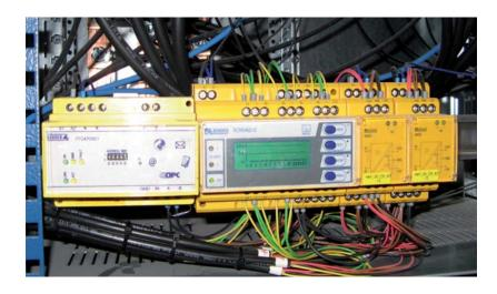
ty technology in the form of AC/DC sensitive residual current monitoring from Bender.
